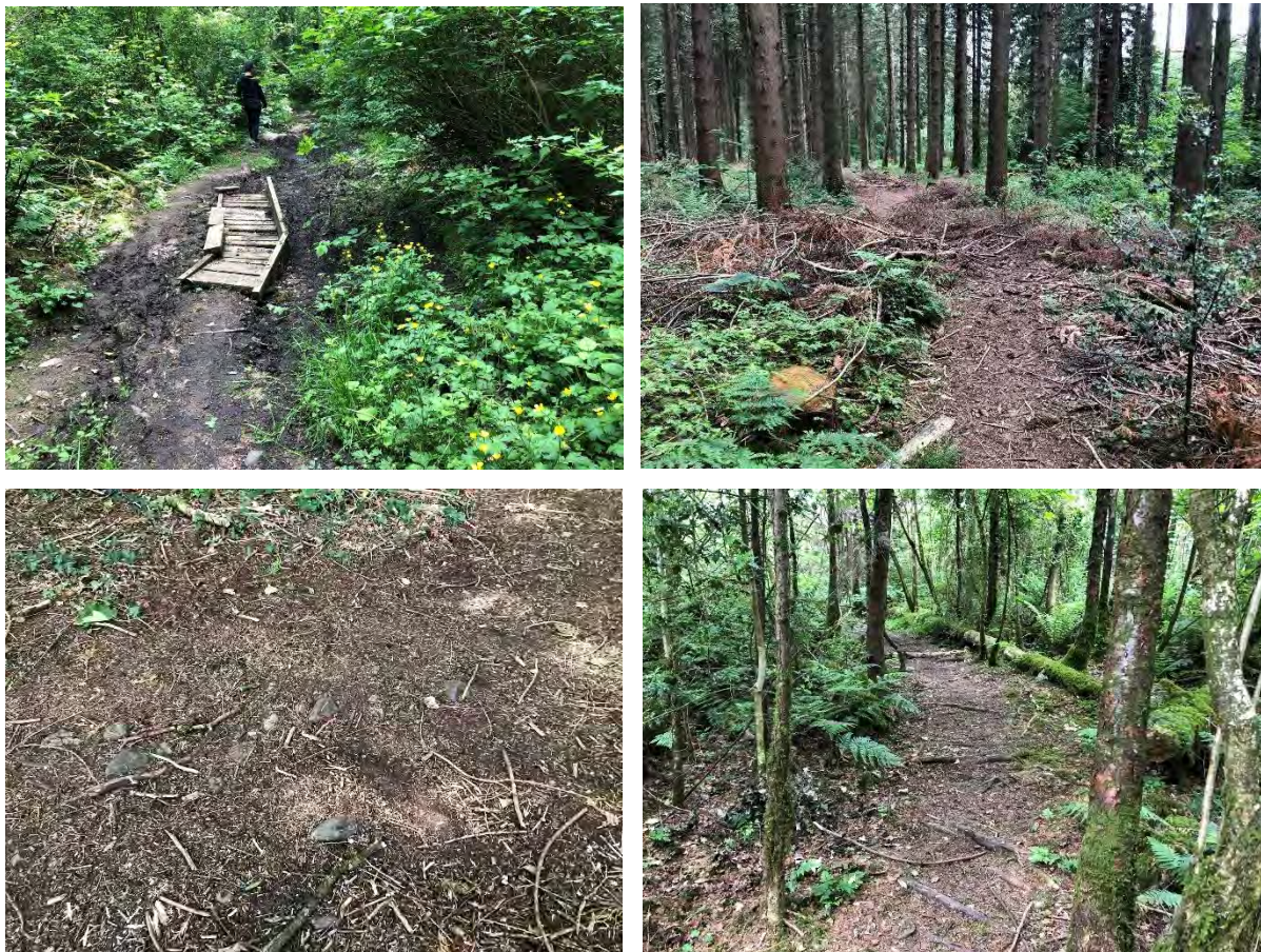
Figure 8 - Clockwise from top left: Poor drainage in occasional spots, poor forestry vegetation clearance, trail surface with tree roots, stone/gravel sub-base across most trails obscured by build-up of organic debris
