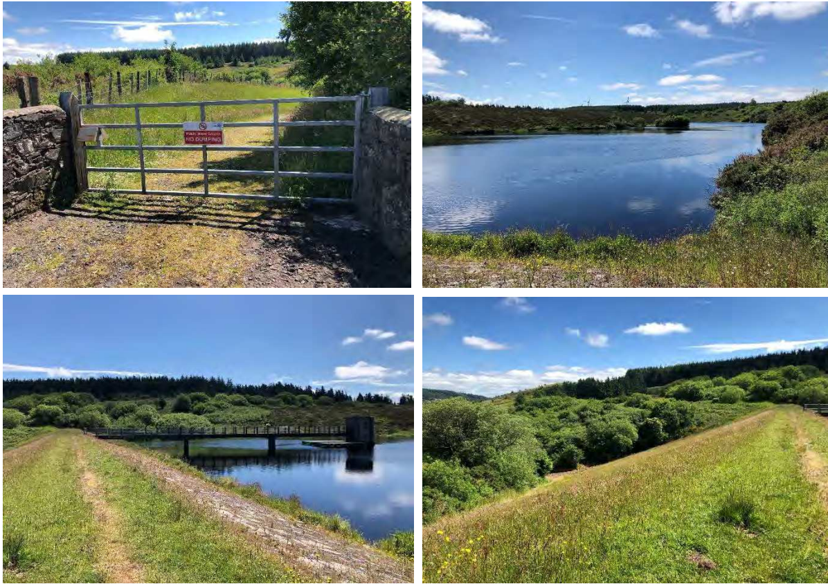
Figure 7 - Eastern extent of the Upper Pond. Clockwise from top left: Steel gate leading to earth dam, View across the Upper Pond towards the west, Downslope of the earth dam, Impounded water level behind earth dam.
