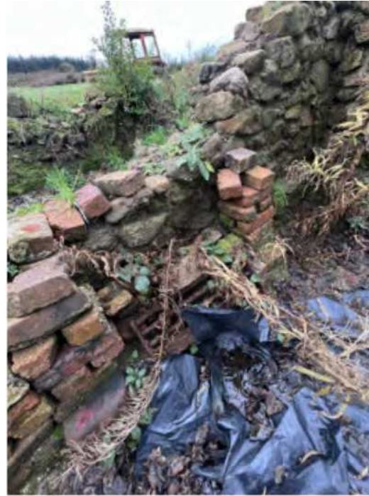
Fig 5 & 6: Photos taken 1 st December 2022 shows the chimney breast in dwellings north gable; and red bricks to a fireplace in the dwellings south gable, respectively. It is unclear if the grate in the second photo is associated with the fireplace. These photos were also taken from within the Planning Statement submitted alongside this application but depict the dwelling on the date of site inspection.
