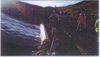
A further layer of Drainage Geocomposite is laid on top of the GCL and covered with 300mm of fine protection layer soil / clay followed by 700mm of sub-soil. On other areas of the cap 100mm of top soil will be added as the final 100mm rather than sub-soil depending on whether the cap is intended to be permanent or intermediate.
