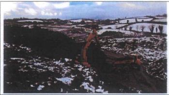
The majority of the soils for the capping works are situated on-site. The photo shows the filling of sub-soil at the sites stockpile area, for use in the regulation layer. 25 Tonne dumpers are used for transporting the sub-soil to the works area.
