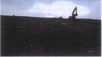
These 2 photos show the sub-soil regulation layer being applied across the works area. A 200mm thick layer is laid to even the surface and prevent damage to the geotextile layers above. The sub-soil is levelled using a bulldozer and 27 Tonne excavator.
