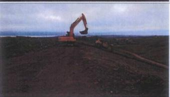
Following placement of the regulation layer 2 layers of geotextiles are laid on top. The picture shows the first layer of Geosynthetic Clay Liner (GCL) being placed and will eventually tie into the anchor trench surrounding the site.
