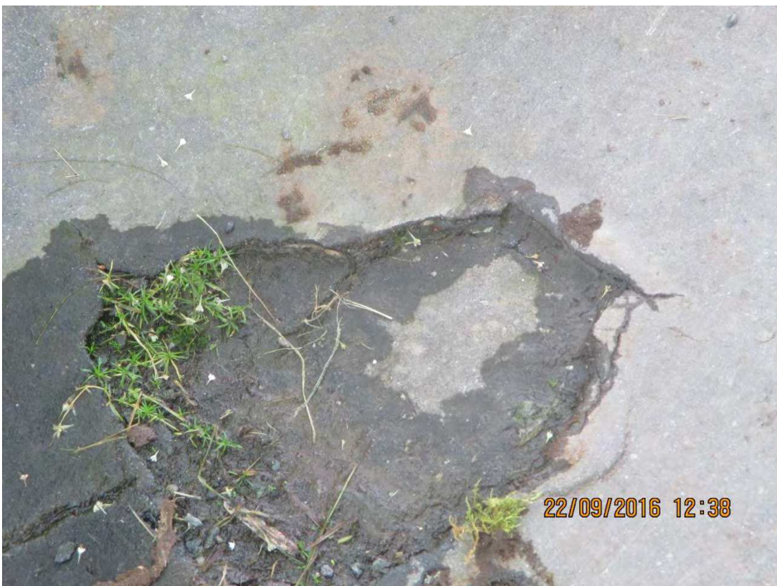
Photograph 66: Surfacing Damage.
