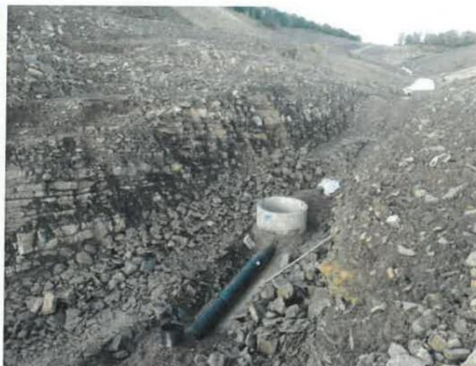
Picture showing the drainage layer geocomposite placed over the top of recently laid GCL and the application of a 300mm deep layer of protection material (left). Picture showing the drainage line / manholes from the unlined Cell 4 and the settlement pond / discharge point (right).
