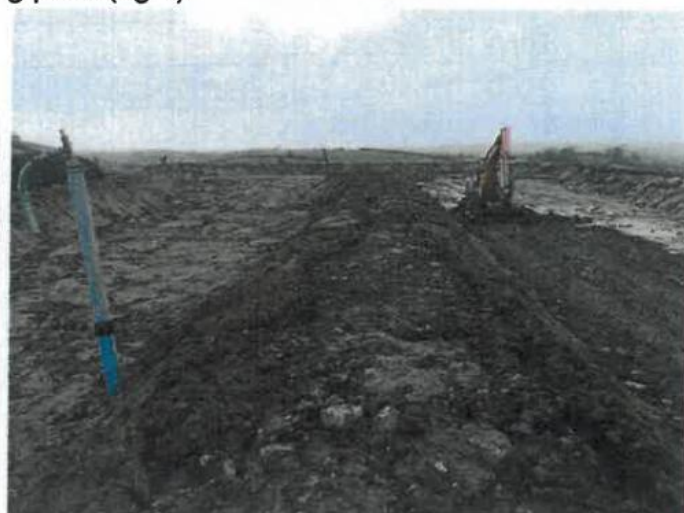
Picture showing stabilised area after the cement has cured (left). Picture showing the construction of the wetlands on top of the stabilised area (right).
