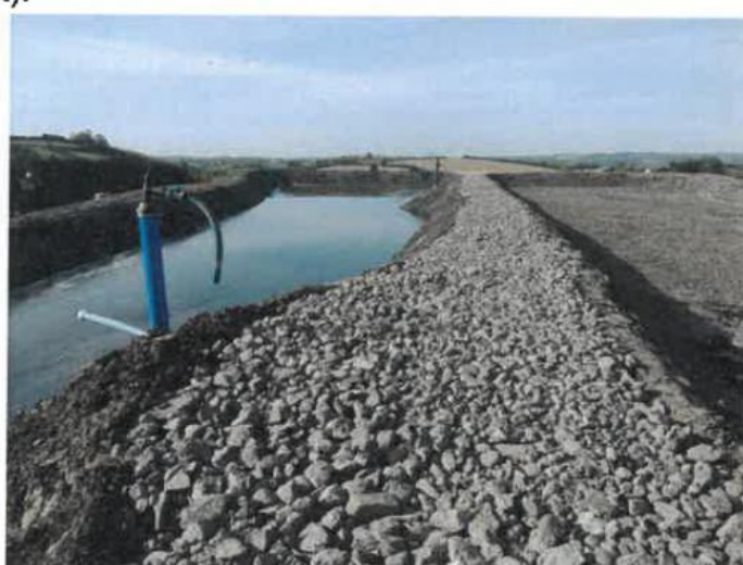
Picture showing the finished cap and access road (left) and the new Integrated Constructed Wetlands (right) showing them being initially filled, with approx. 300mm of water, following planting.
