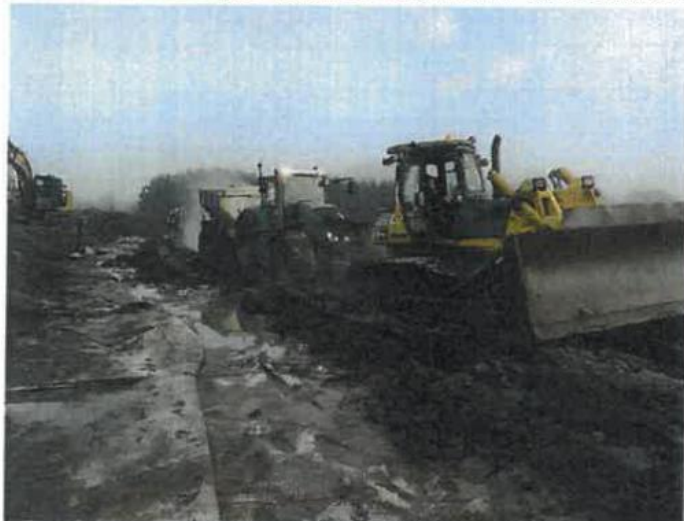
Pictures showing the stabilisation works with the application of cement powder (left) and the mixing with the regulation soils using a specialised blending plant (right).
