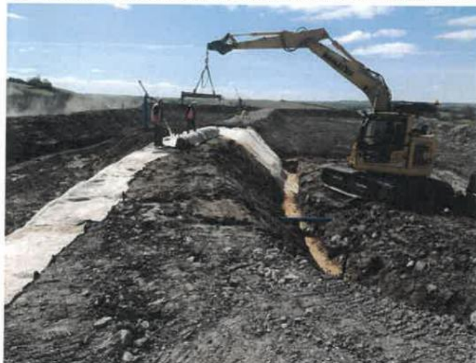
Pictures showing the lining of the wetlands central bund (left) and the finished cap and perimeter drainage system adjacent to the main office (right).
