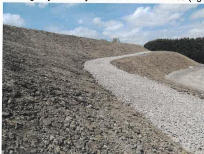
Picture showing the finished cap and access road (left) and the new Integrated Constructed Wetlands (right) showing them being initially filled, with approx. 300mm of water, following planting.
