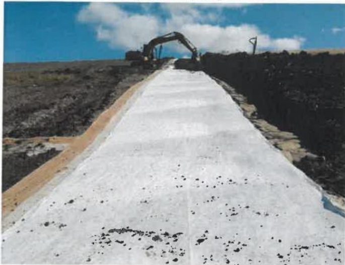
Picture showing the drainage layer geocomposite placed over the top of recently laid GCL and the application of a 300mm deep layer of protection material (left). Picture showing the drainage line / manholes from the unlined Cell 4 and the settlement pond / discharge point (right).
