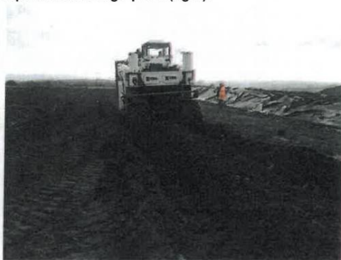
Pictures showing the stabilisation works with the application of cement powder (left) and the mixing with the regulation soils using a specialised blending plant (right).
