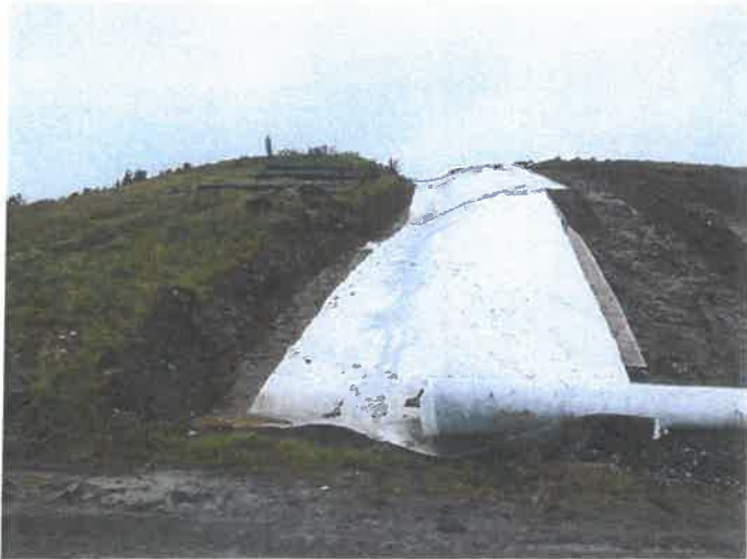
Pictures showing the drainage layer geocomposite placed over the top of recently laid GCL and the application of a 300mm deep layer of protection material.
