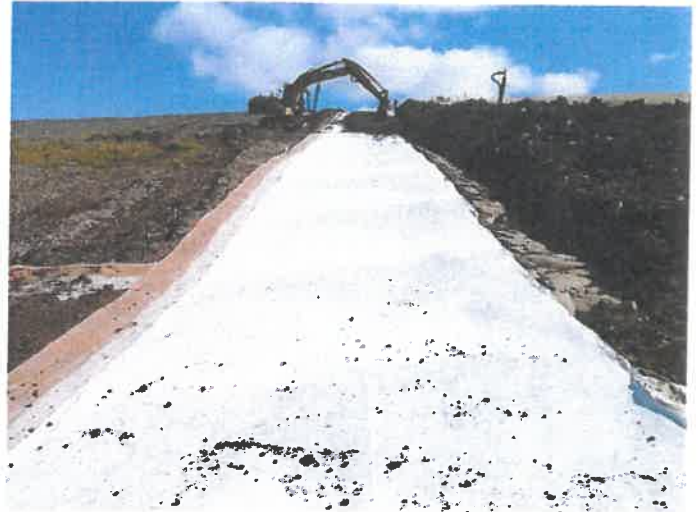
Pictures showing the drainage layer geocomposite placed over the top of recently laid GCL and the application of a 300mm deep layer of protection material.
