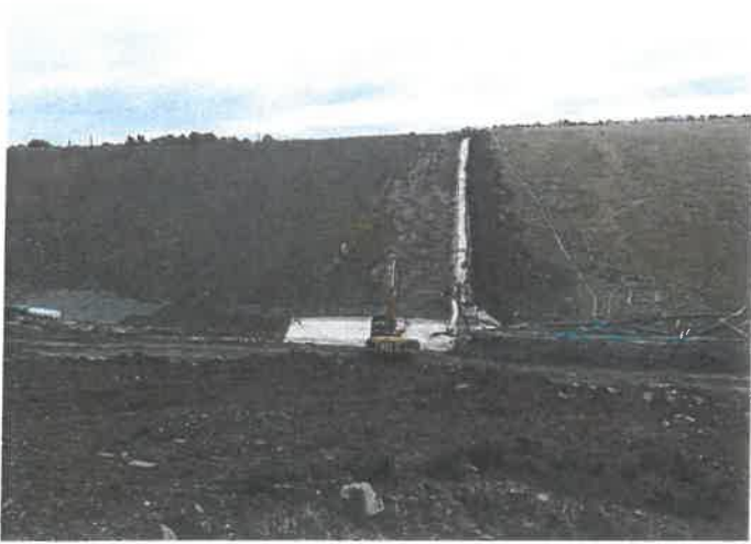
Pictures showing the stripping back of restoration soils from existing cap to expose the GCL layer and then the application of GCL to Phase 4 with a 300mm overlap.
