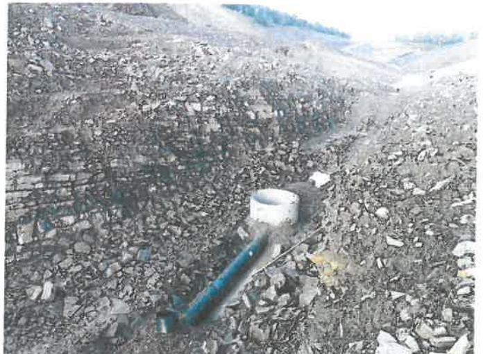
Pictures showing the installation of drainage between the Phase 4 cap and the existing wetlands (left) and the drainage line / manholes from the unlined Cell 4 and the settlement pond / discharge point (right).
