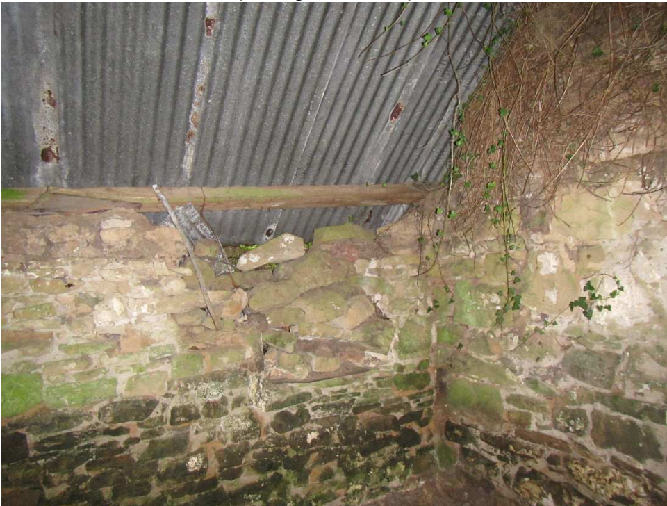
Rear wall with window opening blocked up
