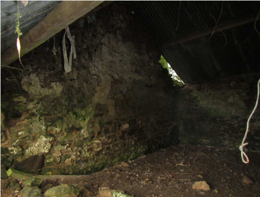
Rear wall with window opening blocked up
