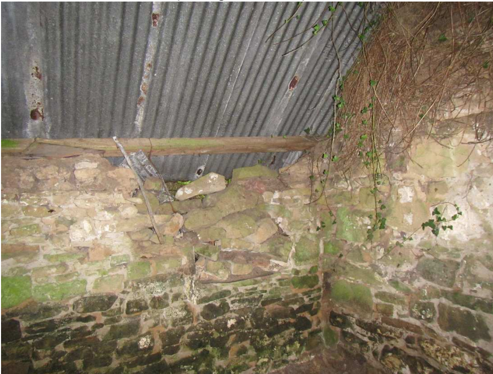
Rear wall with window opening blocked up
