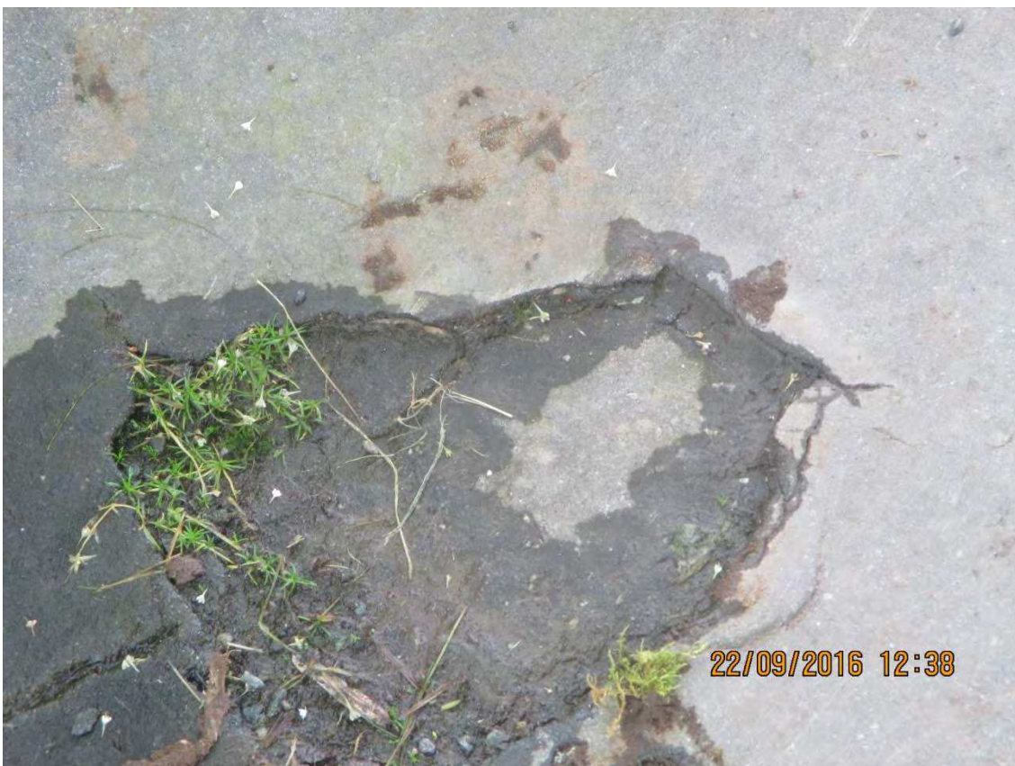
Photograph 66: Surfacing Damage.
