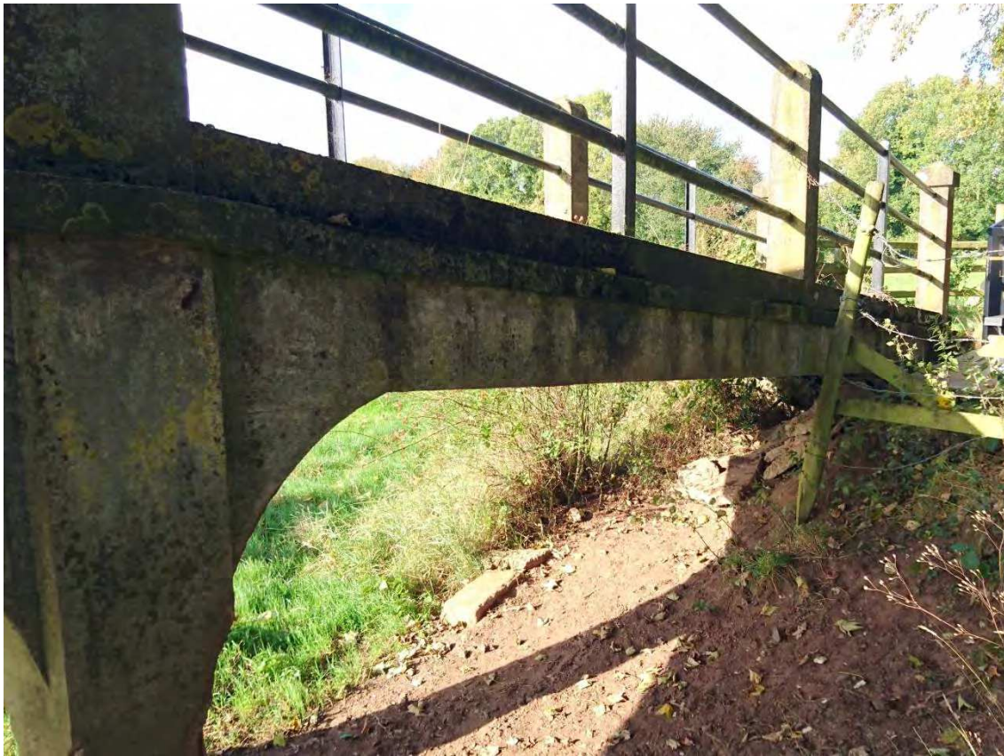
Photograph 15: D/S Edge Beam
